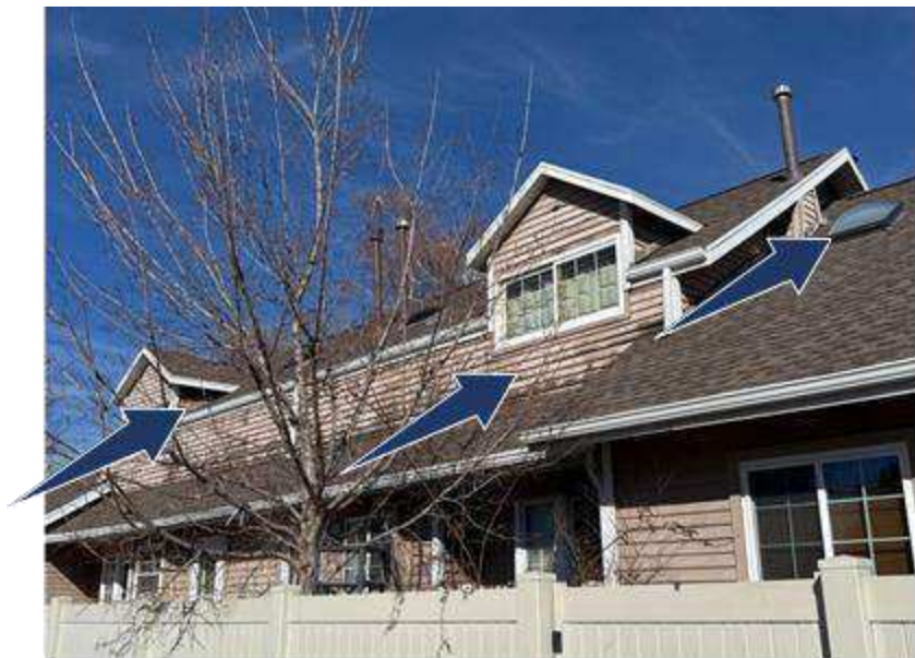
Building 15 South Side
