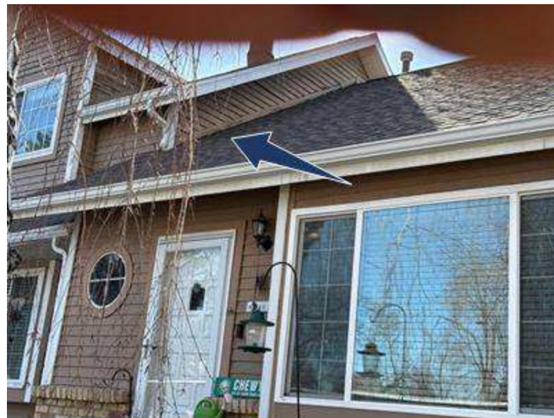
Building 15 North Side
