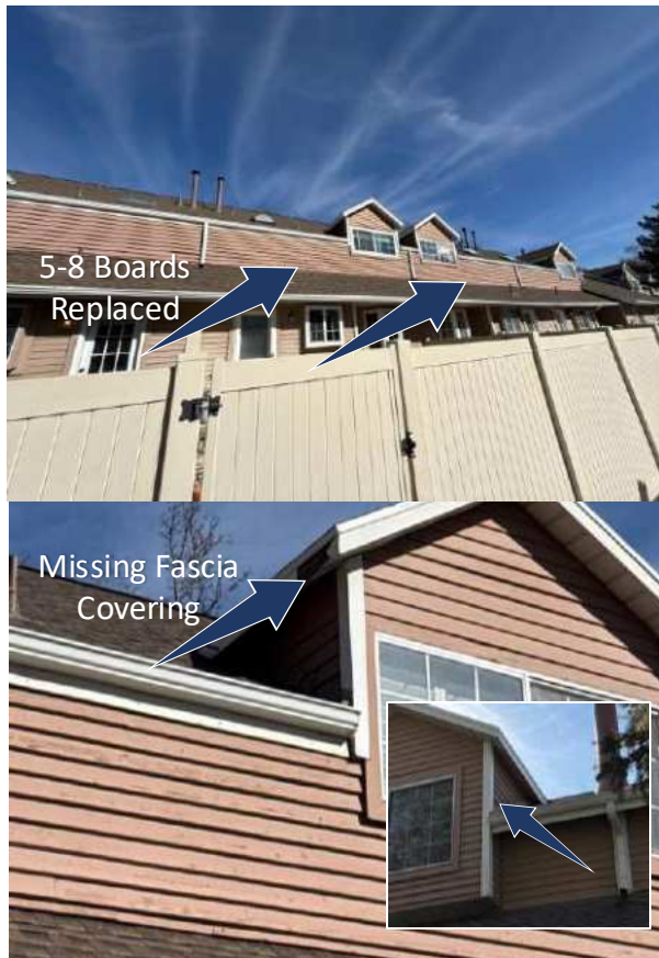
Building 8 South Side
