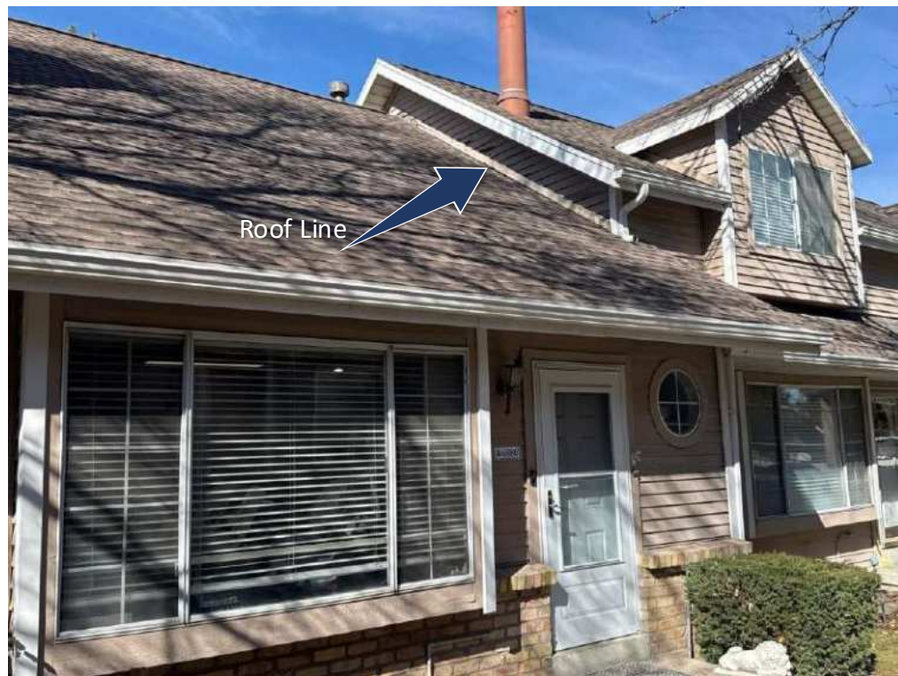
Building 11 South Side
