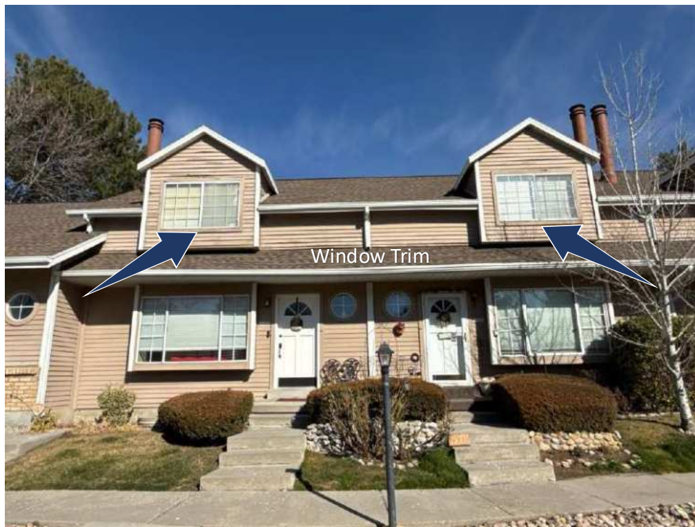
Building 12 South Side
