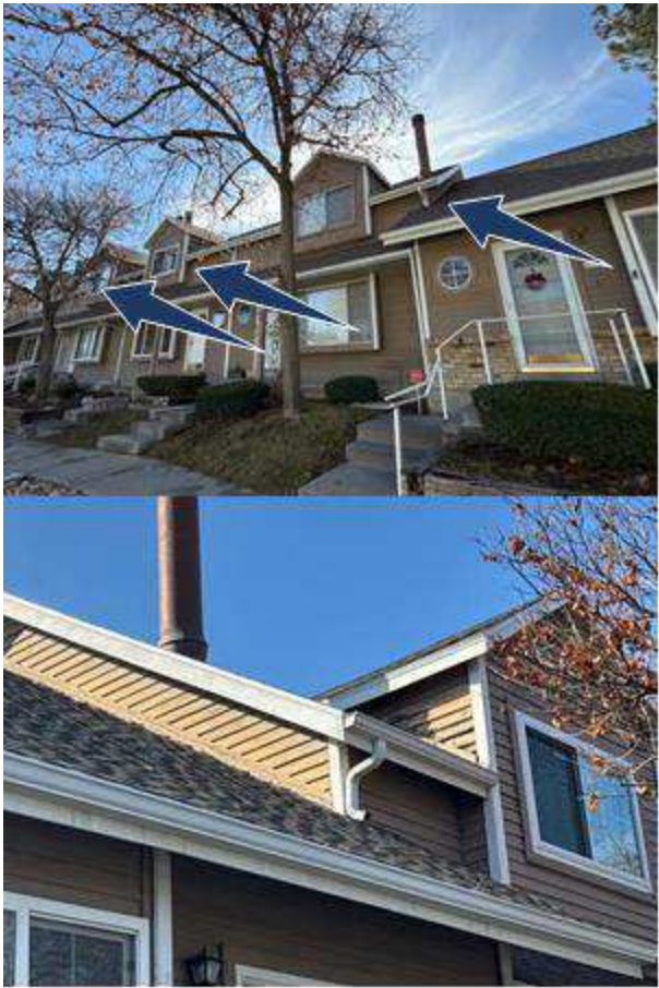
Building 14 North Side
