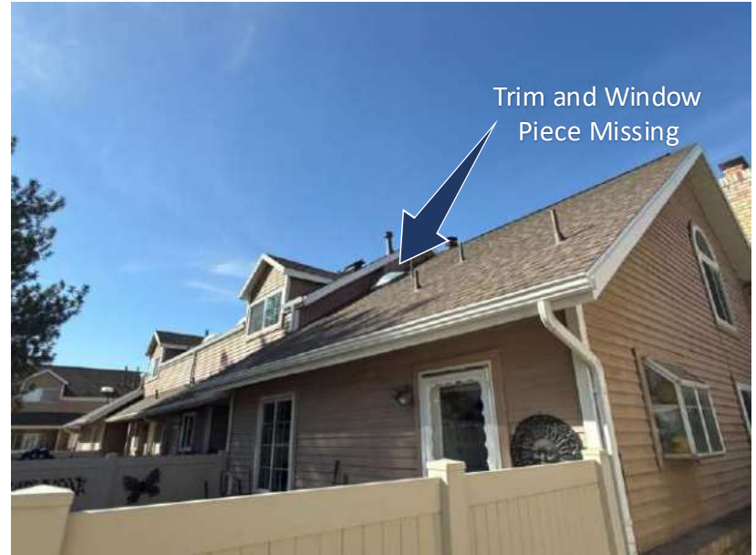
Building 13 East Side
