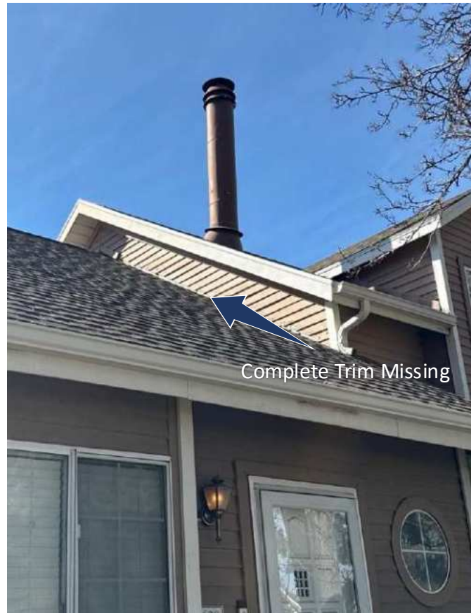
Building 8 North Side
