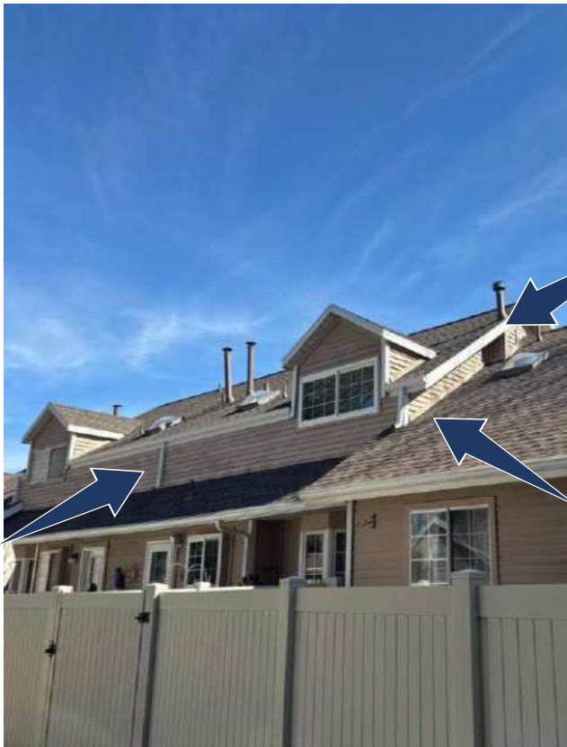
Building 5 West Side
