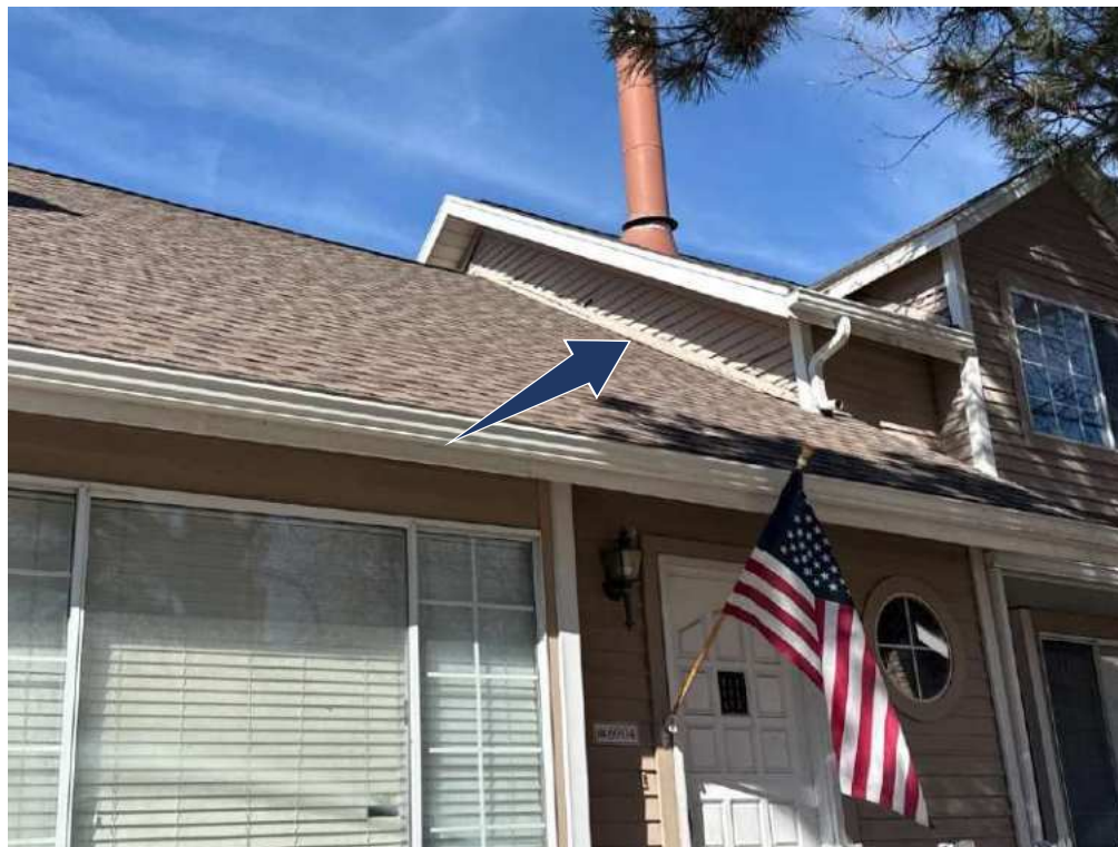
Building 10 East Side Garage Area
