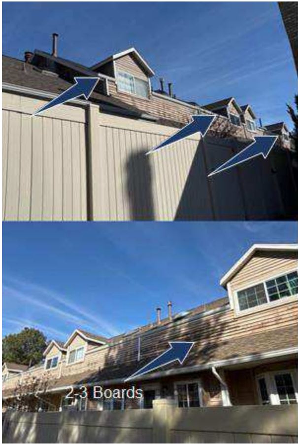
Building 14 South Side
