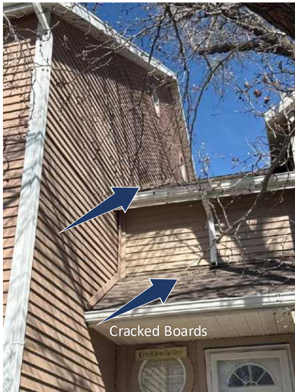
Building 4 South Side
