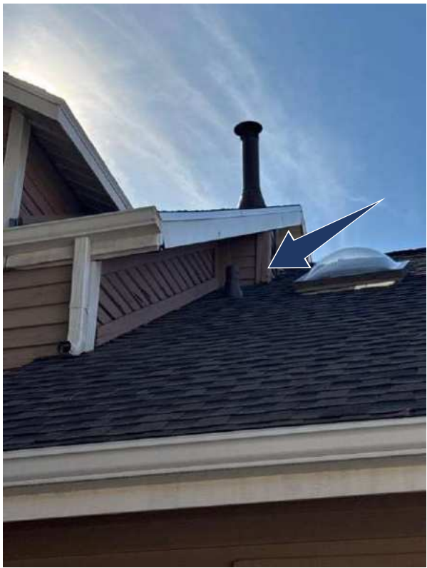
Building 4 North Side
