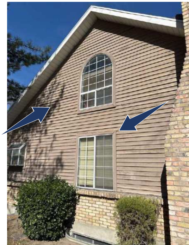
Building 1 South Side
