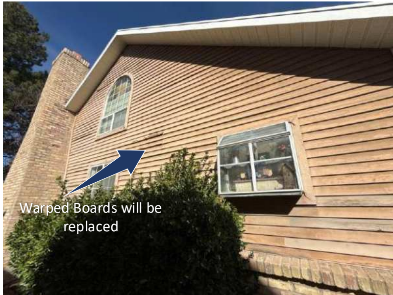
Building 13 South Side
